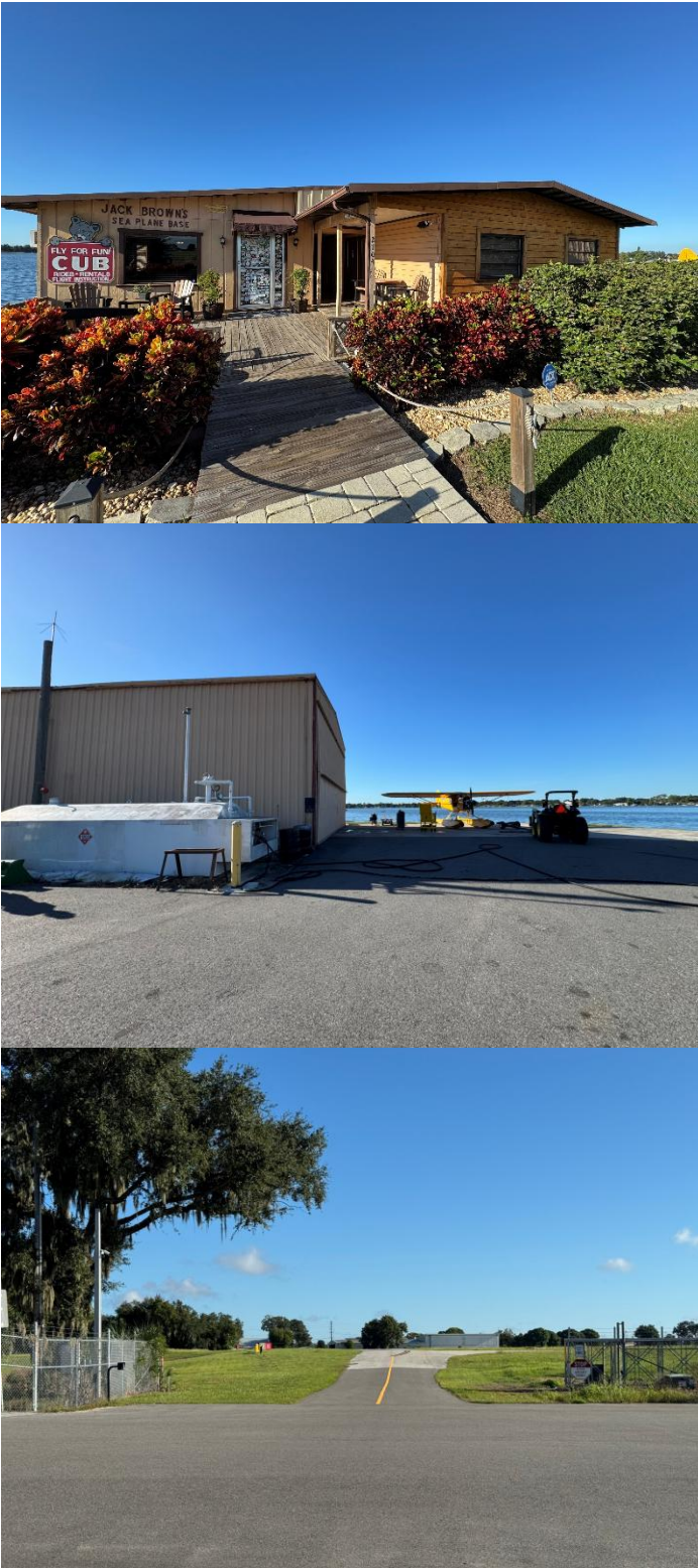
FIGURE 1.29: JACK’S SEAPLANE BASE FACILITIES
