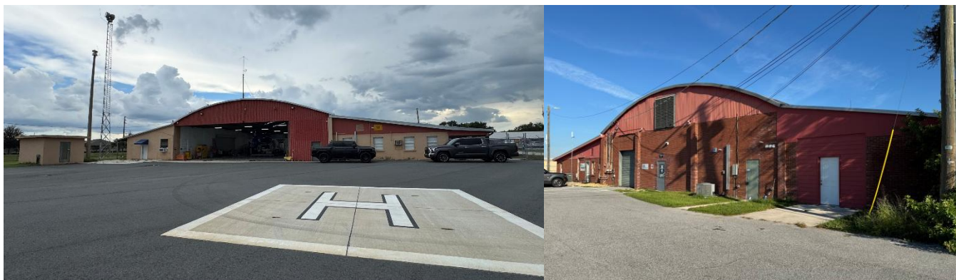
FIGURE 1.21: BUILDING 10 EAST AND WEST SIDES
