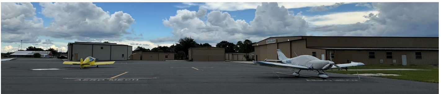
FIGURE 1.19: SOUTH APRON WITH BUILDINGS 105 AND 110
