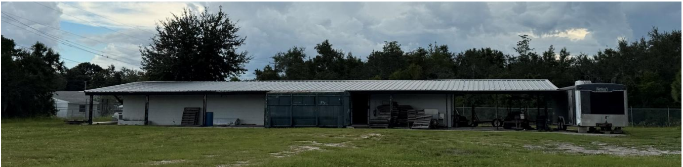
FIGURE 1.22: BUILDING 900 – RECORDS STORAGE
